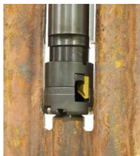
Remove membrane from between tubes
