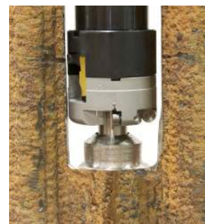
Remove membrane and overlay/cladding from between tubes
