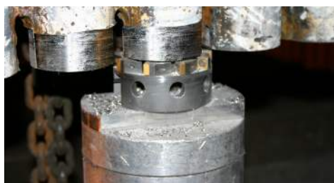
Overlay is removed from new and existing tubes and their ends are prepared for welding to new tubes.
