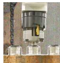
Boiler tube membrane overlay removal and bevel.
